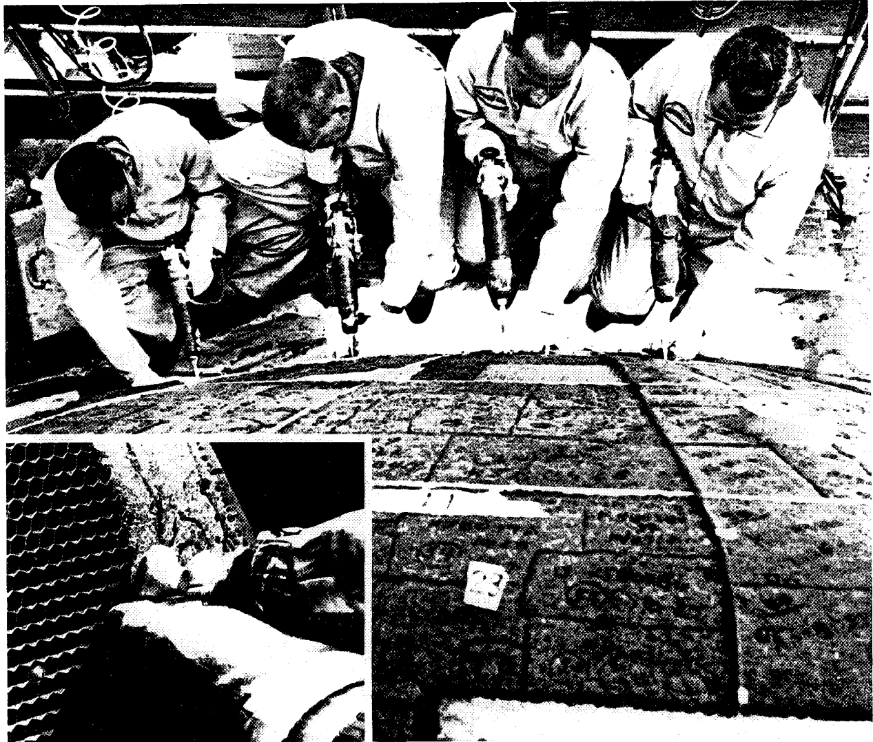
Special ablative material is injected into each cell of heat shield by technicians at Avco plant in Lowell, Mass.
